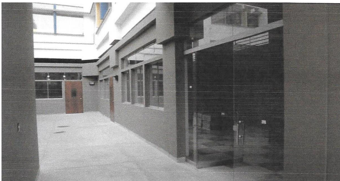
Vista interior FAING (Bloque 1)
